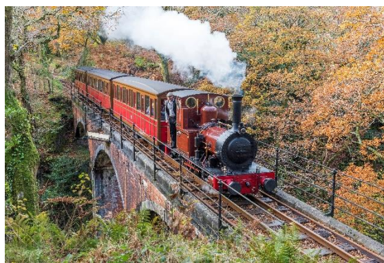
Talyllyn Railway crossing Dolgoch viaduct (Component Part 6) © Rheilffordd Talyllyn Railway
